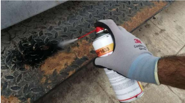
Cleaning with 1633 Rust Remover
