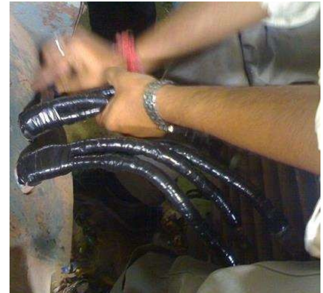
Properly insulated and mechanically protected motor lead wires / cables
