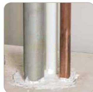
Firestops service penetrations passing through fire-rated floor or wall assemblies.*
